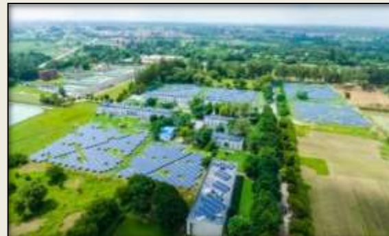
2000 kWp Solar Plants on Under Ground Water Tanks in Sec 39
